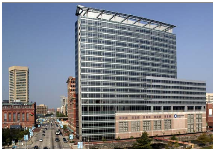
One of Maryland's main electricity distribution companies is Baltimore Gas & Electric (headquarters shown here), which plays an important role in advancing retail competition by connecting competitive electricity providers to homes and businesses in its area.
