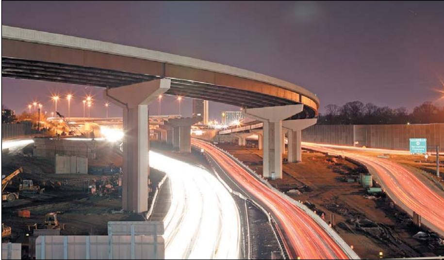
High occupancy toll (HOT) lanes are proposed for Interstate 495, extending 12 miles from west of the Springfield Interchange pictured here.
