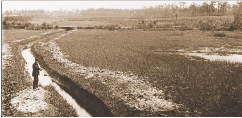
The chief field agent for the American Red Cross, Dr. Hubbell, looks over ditches dug by hurricane survivors. The flooded lands needed to be drained so crops would grow.
