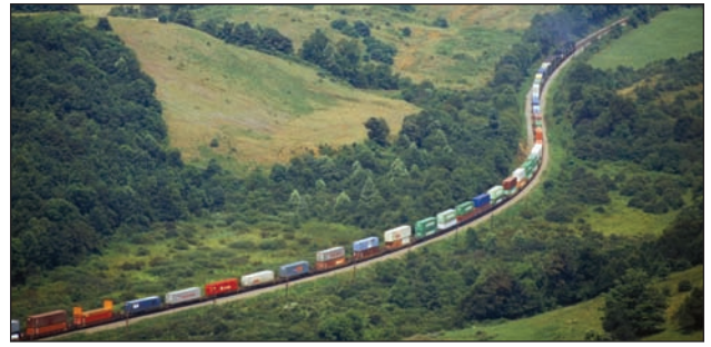
Raising tunnels to accommodate double-stacked containers on trains will move cargo more cheaply and efficiently from Hampton Roads ports to Chicago.
