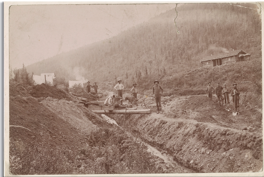
Western gold miners, such as these in El Dorado, Calif., circa 1850, built elaborate ditch systems throughout the countryside to divert water for panning gold and operating mines.
