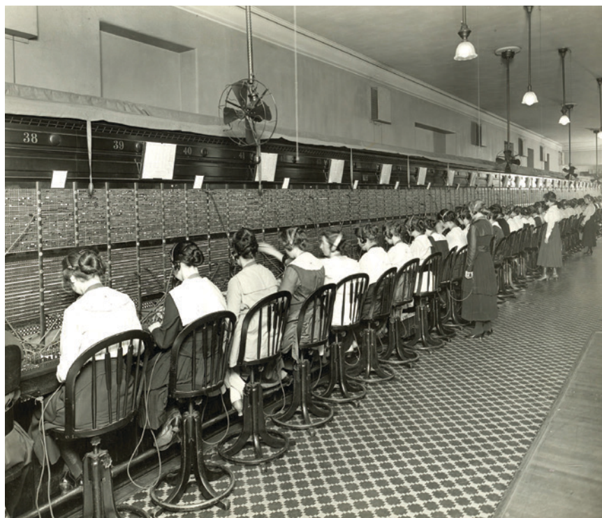
Operators in 1917 at a large switchboard of the New York Telephone Company in the financial district of lower Manhattan.
